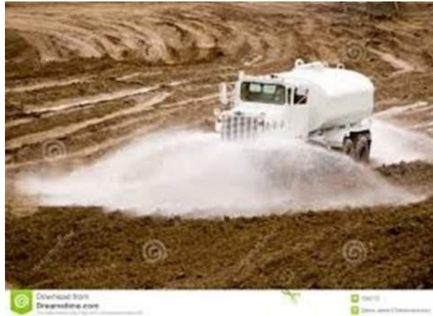
Figure 5.2: Dust Control Water Trucks (Illustrative Only)
